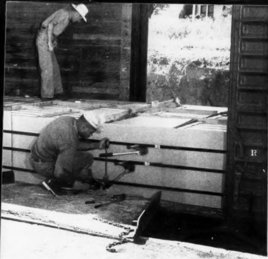
View at left shows the tightening of straps of filled car.
